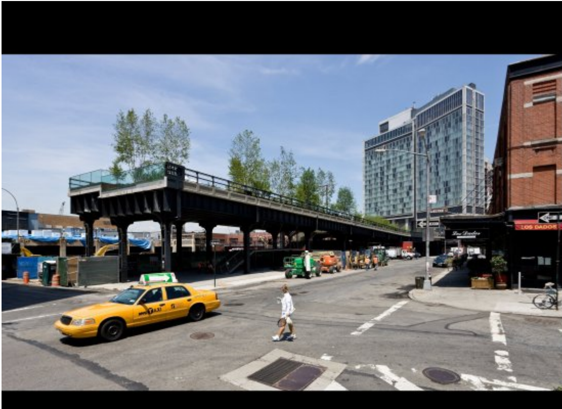
Gansevoort Plaza and Stair, Gansevoort Street and Washington Street, looking North
